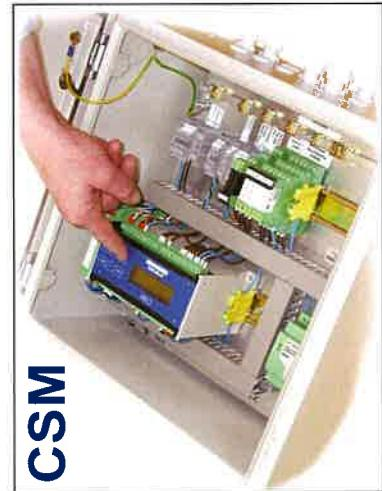
PIAB Crane Safety Monitor (CSM) is an electronic control unit to be used in Overload Protection Systems.
