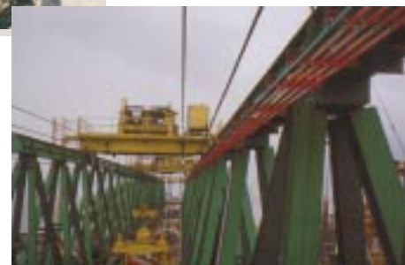
Bridge Construction Crane
